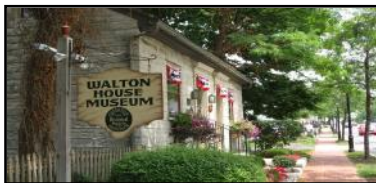
Walton House, Built 1838
